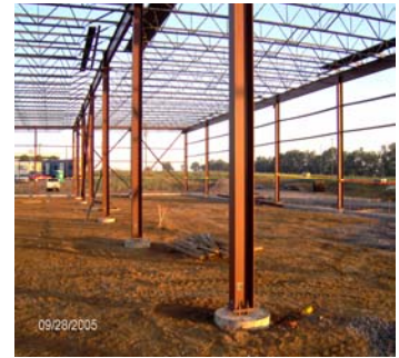
Steel and bar joist installation
