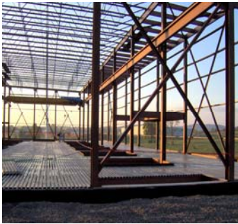
Metal deck prior to concrete
