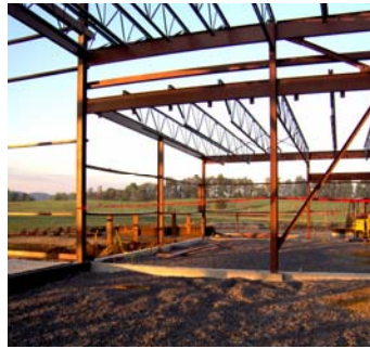
Slab on grade being prepared
